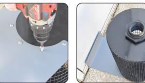
1. Position the support as shown and screw it to the bottom of intake screen. Be careful to not over tighten.
