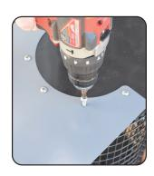
3. Align the remaining support on the intake screen with its foot section against the wall. Secure the support to the intake screen.
