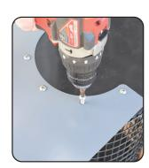
3. Align the remaining support on the intake screen with its foot section against the wall. Secure the support to the intake screen.
