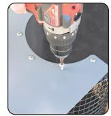
3. Align the remaining support on the intake screen with its foot section against the wall. Secure the support to the intake screen.
