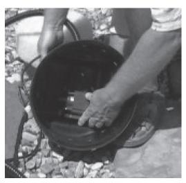
Place pump in bottom chamber of filter. We recommend EasyPro mag drive pumps up to 850 GPH.
