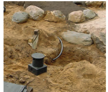
Use leftover dirt from reservoir to build up berm around top of waterfall if needed
