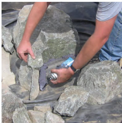
Use EasyPro Black Waterfall Foam to fill in voids between rocks.
