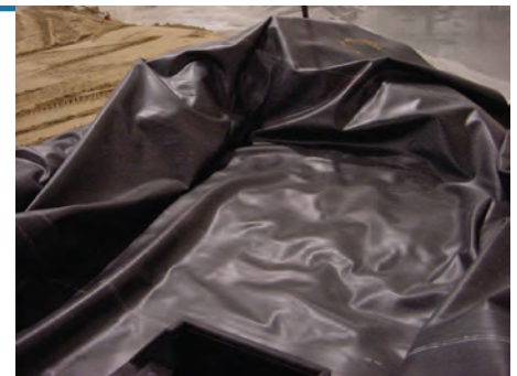
The liner covers the stream bed and goes through the area where the spillway will sit.
