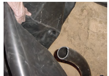
Stretch liner over bulkhead then tighten washer and nut onto bulkhead.
