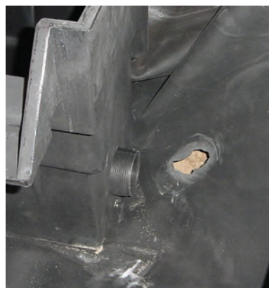
Hold bulkhead up to spillway and cut hole in liner just smaller than bulkhead.
