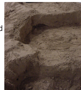
Sculpt and compact dirt in stream area before installing liner
