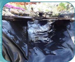
This design technique starts with a valley, right above the bottom drainpipe that runs from the bottom drain to the skimmer. There is a natural slope from the 18 "depth to the 4.5 foot depth, and the opening is wider at the deep end.
