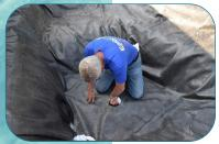
With a clean cloth remove any debris in the drain, on the drain lip, and underside of the liner. This must be clean.
