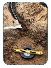
Place and level the bottom drain at the lowest point in the pond. It is best to provide a slight slope in the floor of the pond towards the bottom drain. Trench the tubing below grade and run to the skimmer box location.
