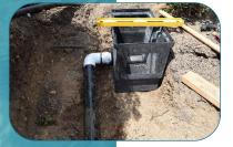
Using a bottom drain kit, connect the tubing, usually to the front of the skimmer box. Although in this application it was connected on the side panel.
