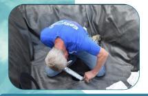
Apply silicone to the top of the bottom drain face place. Cover screw holes and along the inner edge to insure a good seal.
