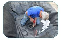
You may use a power tool to start the screws but do not tighten yet. Alternate starts. 12-6, then 3 - 9. Then the rest.
