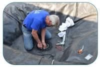
Trim excess liner inside the ring. Apply a final coating of silicone on the edges and wipe smooth.
