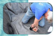
With one hand locate the inner edge of the bottom drain. Then using scissors cut slits from the center to the inner edge.
