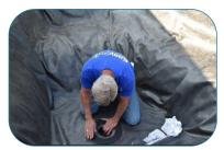
Center ring and line up with screw hole guide marks. Press firmly to spread silicone evenly. Excess should squeeze to all edges.
