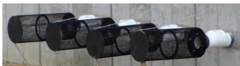
Four PIF8 Intake Filters used to create a 5000 gpm waterfall
