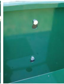
6. Tighten lag screws inside the cabinet. Second person may be needed to support cabinet during this step.
