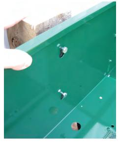
Carefully open cabinet and hang on the installed hex head lag screws.
