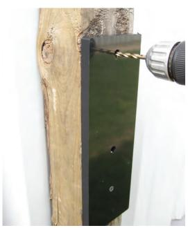
3. Drill <sup>3</sup>/<sub>16</sub>" pilot hole for supplied hex head lag screws in post using holes in the mounting bracket as a guide. Be sure to center the pilot hole in openings on mounting bracket.
