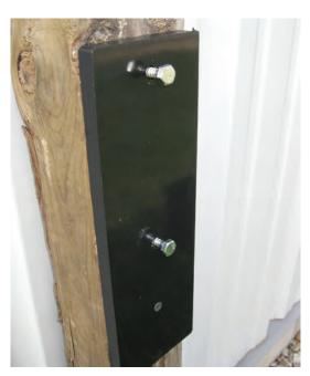
Insert and thread supplied hex head lag screws into drilled holes using a <sup>7</sup>/<sub>16</sub>" wrench or socket. Do not tighten bolts all the way. Leave them approximately <sup>3</sup>/<sub>4</sub>" out.
