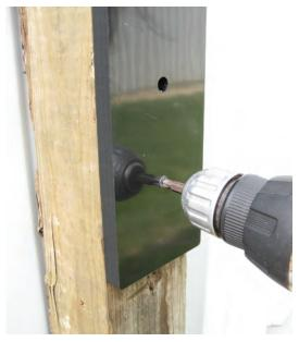
1. Ensure that post is plumb and properly secured or installed to handle weight of cabinet and its contents.
