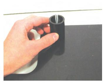
3. Place the spacer blocks over top of each bolt.
