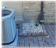
A 1000 gallon system was installed under a future patio area in this backyard setting. The 6' x 11' reservoir area was reduced to only a 24" diameter visible area. The pump controller will be re-plumbed under the patio when completed, leaving no sign of the system!
