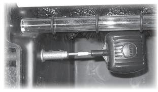
WFS37 — Install the autofill in the back wall of the skimmer by drilling a <sup>3</sup>/<sub>4</sub>" hole 3" down from the top of the skimmer. The auto fill is usually located in the back wall of the skimmer in the pump chamber (see photo).
