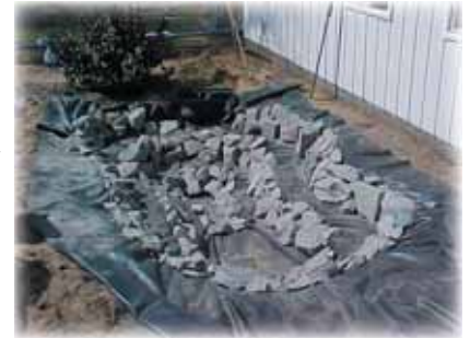
When placing rocks — start in the middle and work outward.
