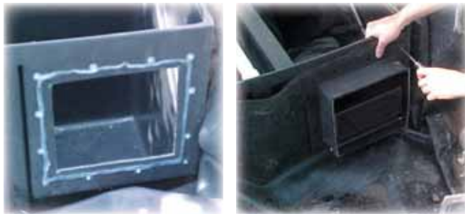
Be sure to use a large bead of silicone around opening. Hold face plate in place and line up holes with an awl. Insert bolts through holes and secure with nut on inside of skimmer.
