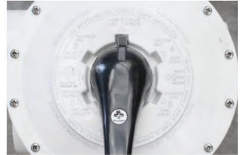
2. Rotate the control handle to “WINTER.” This will allow water to drain from the valve head.
