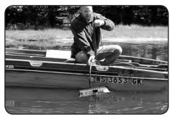
9. Use rope looped around diffuser to assist lowering assembly to pond bottom.
