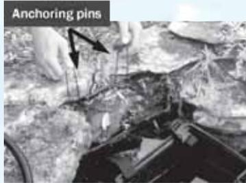
Secure skimmer with straps by threading through slots in back of skimmer and through the anchoring pins that are set 6" - 12" away from pond edge behind liner.
