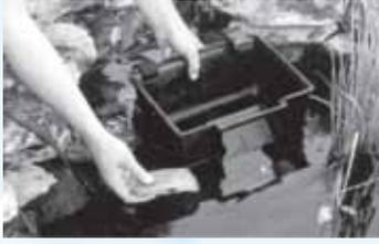
Set skimmer and pump on plant shelf, check for correct height. If the skimmer is too low, you may have to use flat stones or brick to correct the height. Ideal water level should be 2/3 up weir window.
