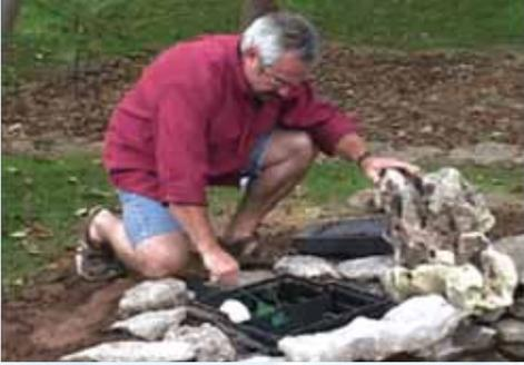
Shut off pump prior to cleaning skimmer. Remove the cover to expose the clean out area.
