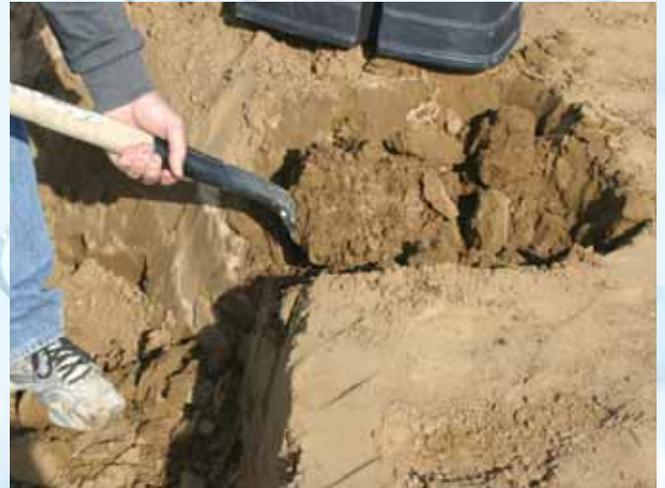
Dig a pocket for the skimmer on the edge of the pond. Over dig the pocket by at least 4" in all directions to ensure plenty of room for the skimmer.
